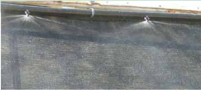
Modular half-circle sprayer 100 l/h mounted every 1.0 m
