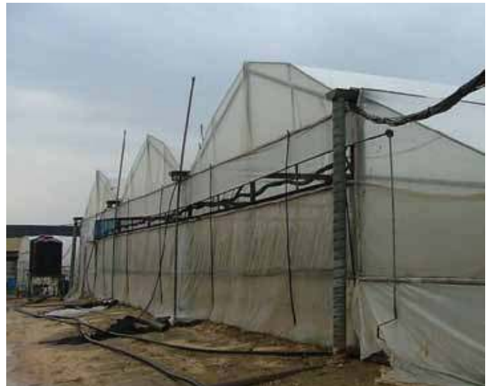
Tomato greenhouse, Mamkad 16 sprinklers on the roof along the gutters
